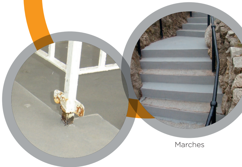
Garde-corps descellés
