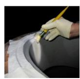
High temperature vessel suffering from severe corrosion. Pitted surface rebuilt using with Belzona 1511.
