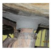
Process kettle developed holes in the weld seam as a result of corrosion. Belzona 1511 used to repair holes for the long term.
